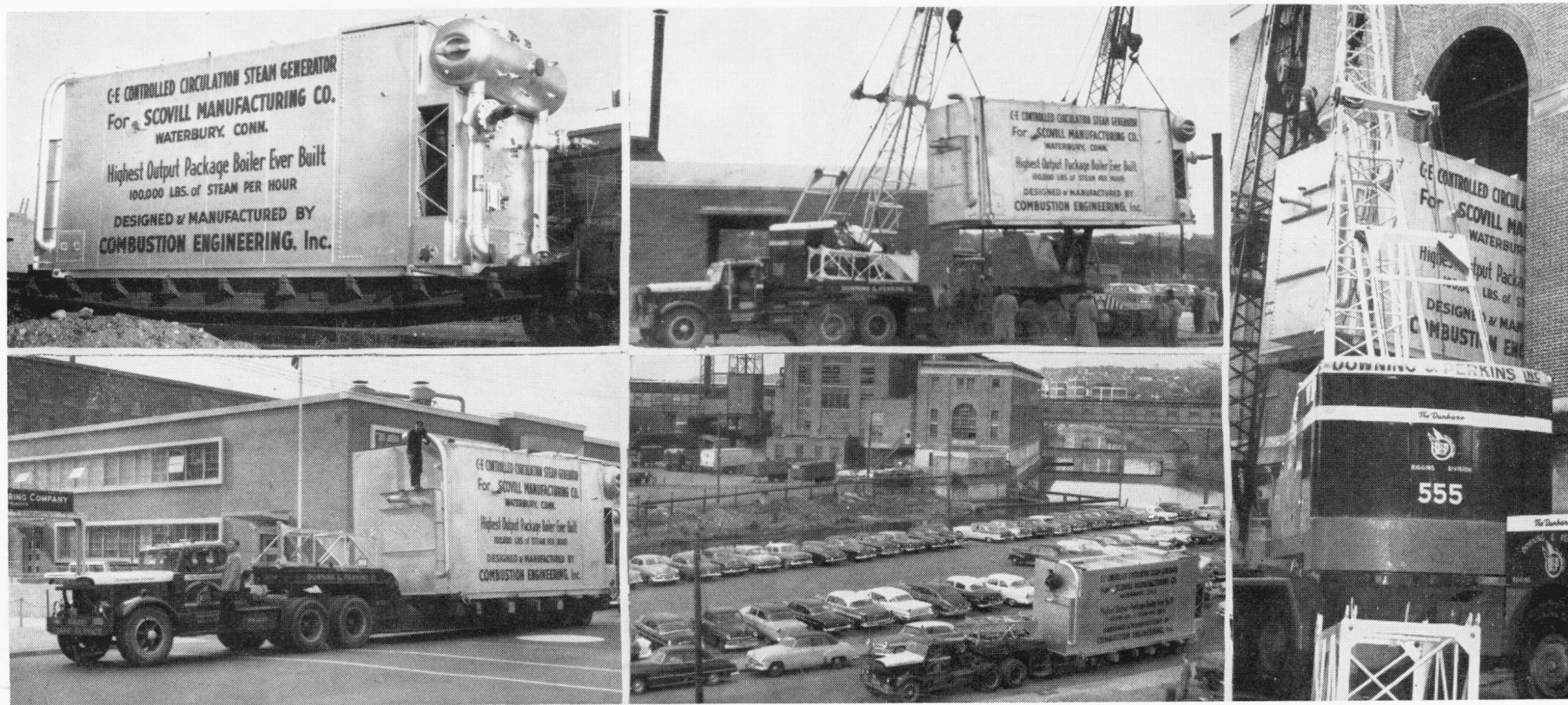
Arriving at its destination is this new 65-ton boiler which is being installed in the Steam Department. Coming by rail from St. Louis, the above photographs
